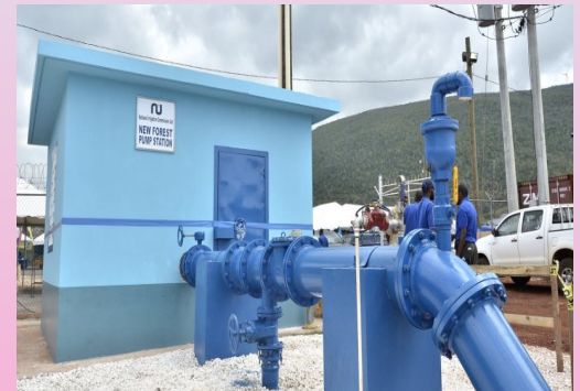
New Forest Pump Station
